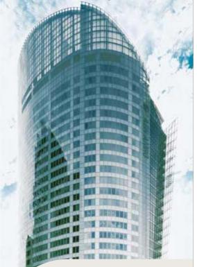
Designed by the architect Renzo Piano, the twin towers of Aurora Place stand out with their deconstructed form. The glass canopy facades use Somfy motor systems so that occupants of the residential part of the building can let fresh air in or keep cold air out, depending on the weather.
