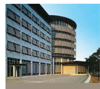
The "live façade" is a membrane, playing host to numerous exchanges between the inside and outside of a building. By reacting in real time to climatic variations, automated solar protection allows for more intelligent, more economical, more aesthetic, and above all, more environmentallyfriendly flow management.
